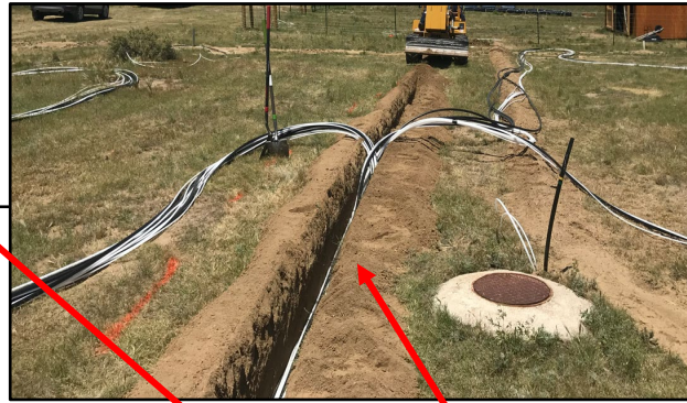
Installation of the subgrade groundwater conveyance network
