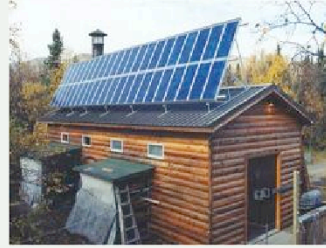
An off-grid, 770-watt PV system at Brooks Camp, AK, powered an air sparging pump used for treating groundwater contaminated by former underground storage tanks.
