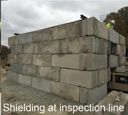
Shielding at inspection line
