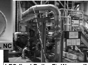
LFG-fired Boiler Ft. Wayne, IN
