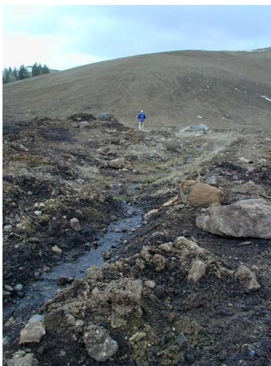
FIGURE 5-3 Seep Observed Near Toe of Waste Rock Impoundment Source: Möller, 2002
