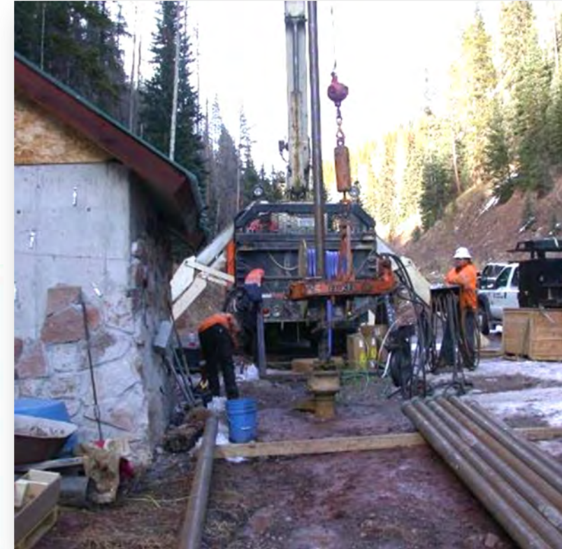
Pump replacement in Liberty Well in September 2018
