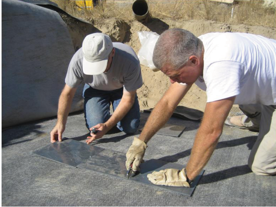
Fig. M. 5. Cutting sample perimeters during GCL exhumation.
