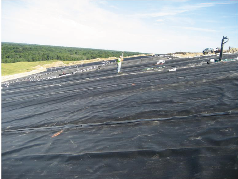
Fig. M. 27. GM overlying GCL before placement of overlying soil layer. Condensation for solar heating was observed underlying.
