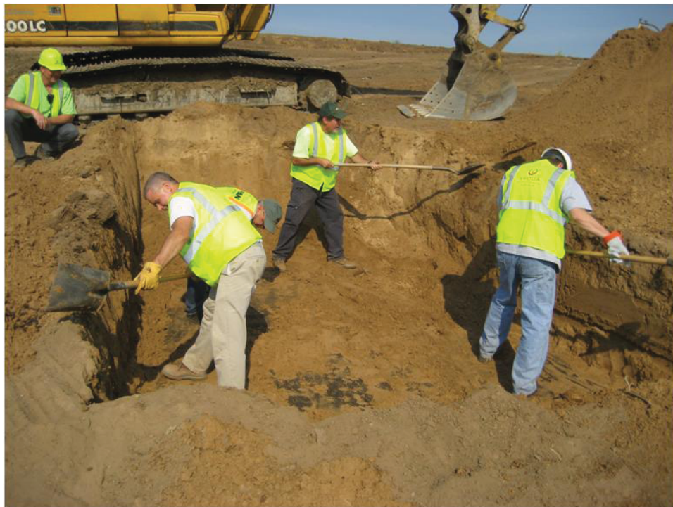
Fig. M. 9. Manual removal of soil layer overlying geocomposite barrier layer.
