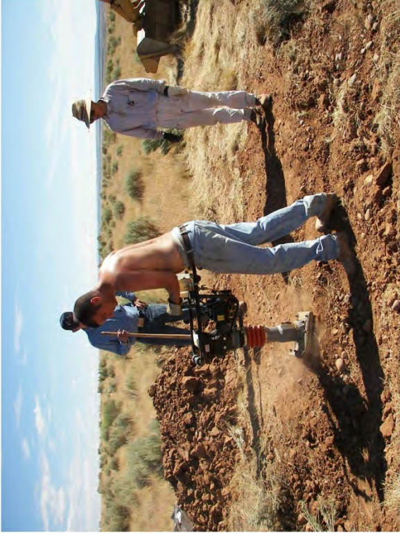
Fig. A.97. Re-compacting soil after sampling.
