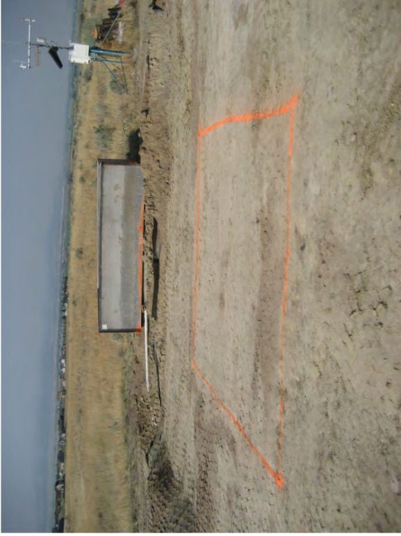
Fig. A.11. Cover soil removed prior to SDRI installation.
