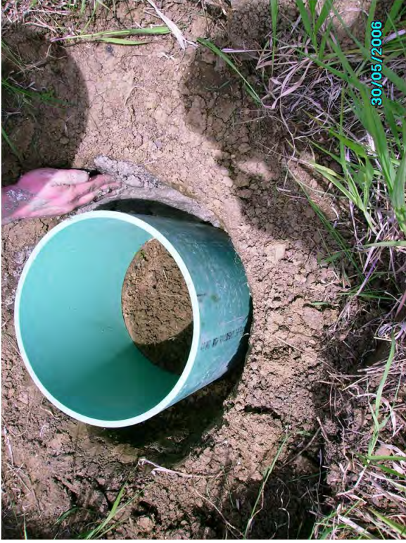
Fig. A.44. Grouting TSB with bentonite paste.
