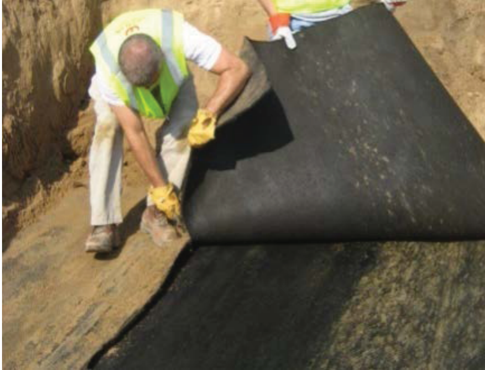
Fig. M. 10. Removal of GDL exposing GM.
