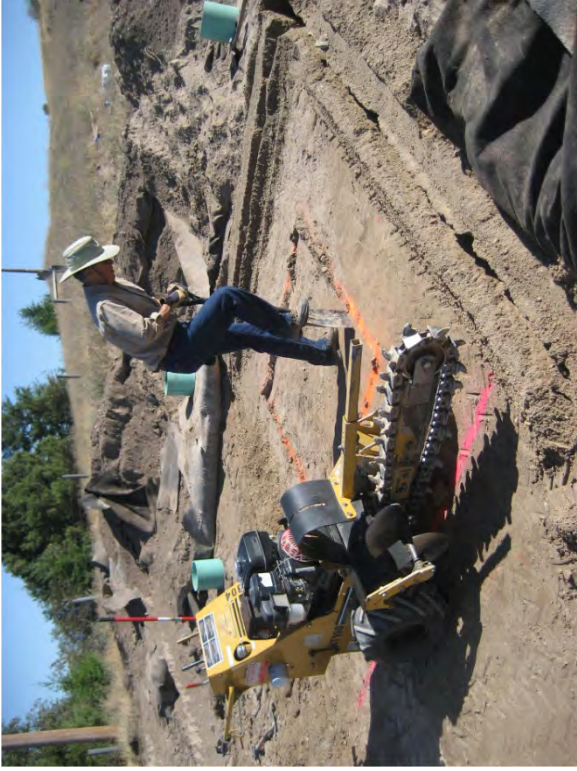
Fig. A.29. Installation of SDRI seating trenches.
