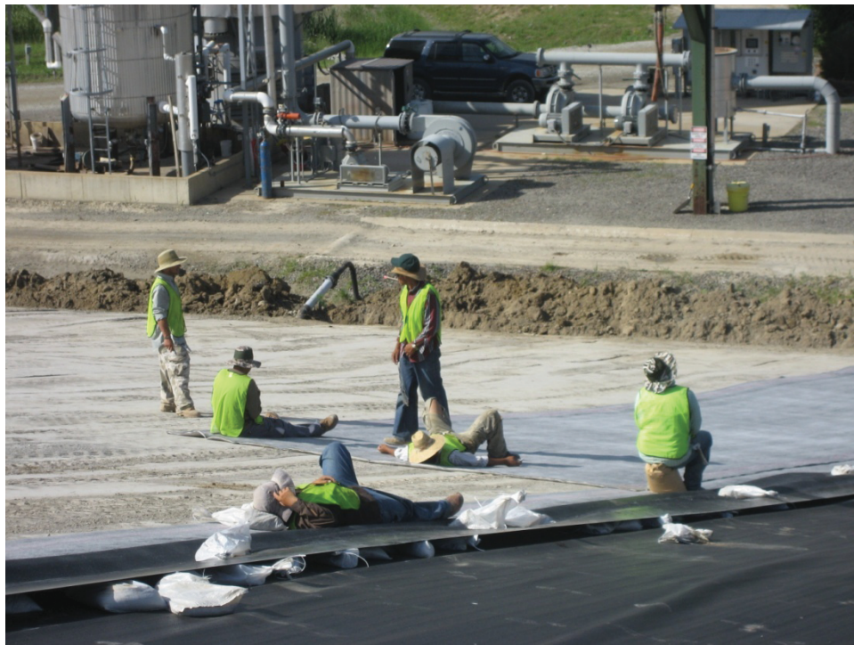
Fig. M. 28. GCL instillation team between rolls.
