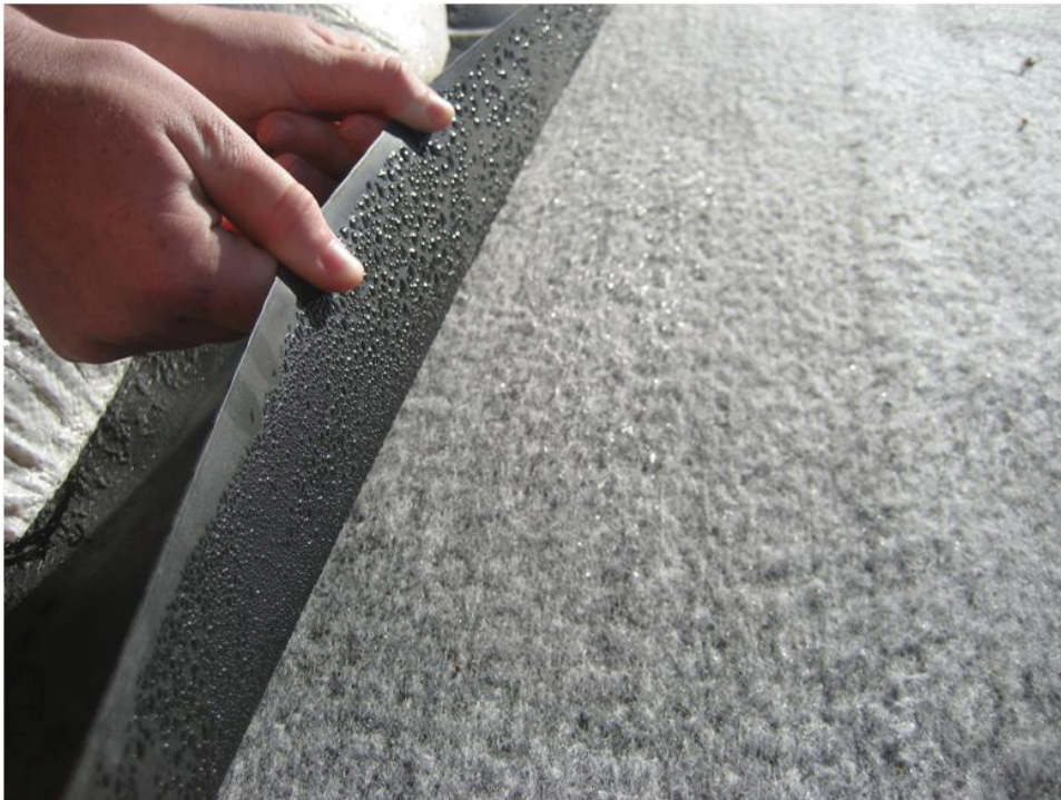
Fig. M. 26. Condensation on GM overlying GCL underside from solar heating.
