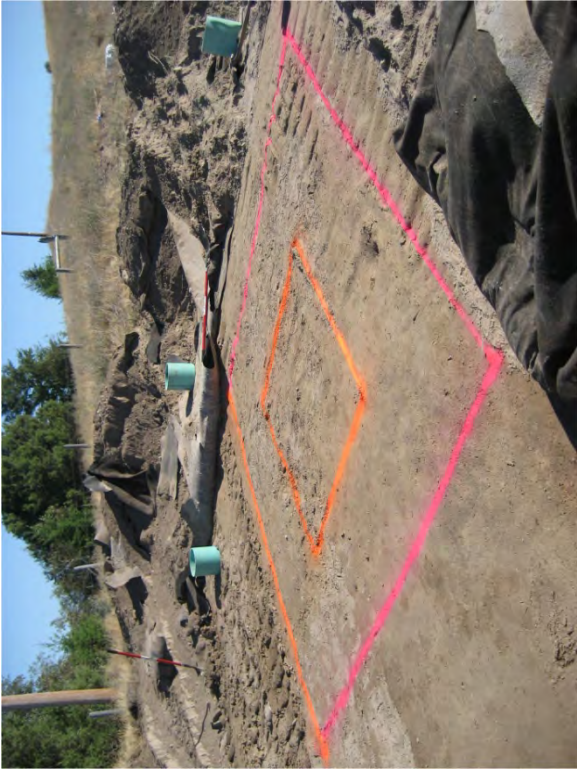
Fig. A.28. Installing SDRI under GM into CCL.
