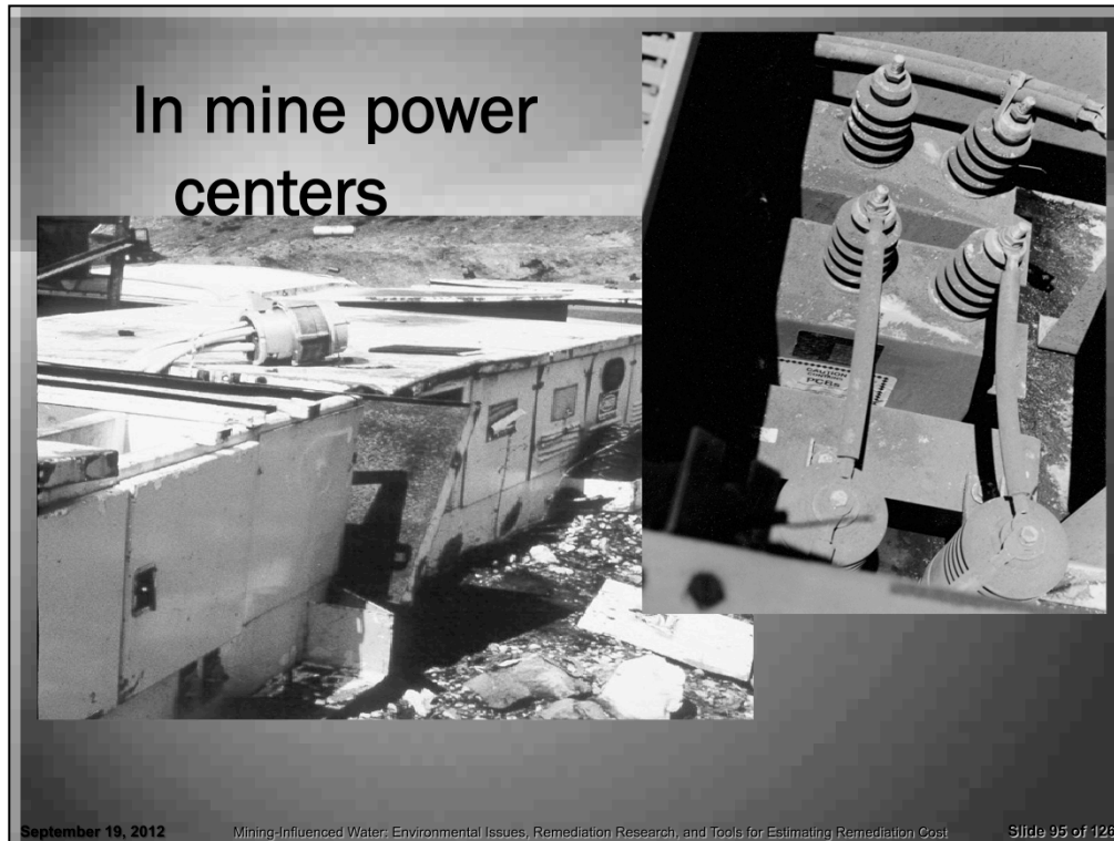
Mine power center with large PCB capacitors awaiting disposal at a Utah coal mine
