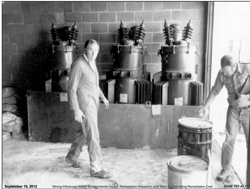
76 gallon Pyranol transformers removed from the 2010 substation now in storage in the surface warehouse.
