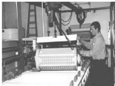
Barrel method electroplating
