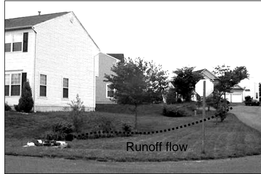
Residential bioretention system
