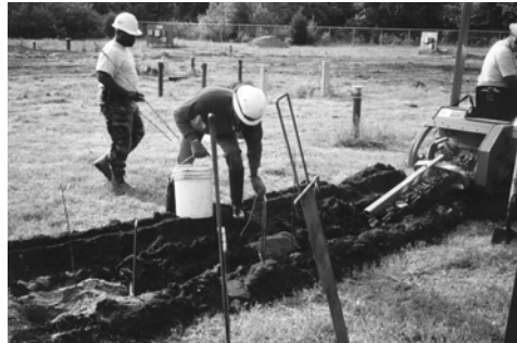
Trenches were dug in the Containment Area. Willow cuttings were deeply planted in backfilled trenches.
