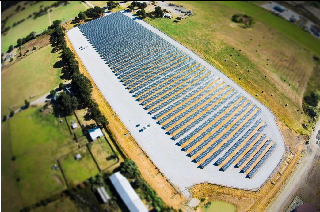
Solar array, Georgia
