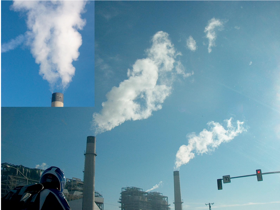
Figure 3.3 Two power plant plumes under the influence of condensation and evaporation physics, leading to the concept of plume concentration contours. Inset: Bifurcating plume exhibiting complex plume symmetry.
