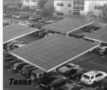
Solar array providing covered parking and power
