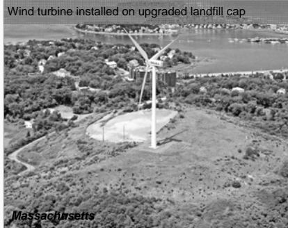
Wind turbine installed on upgraded landfill cap
