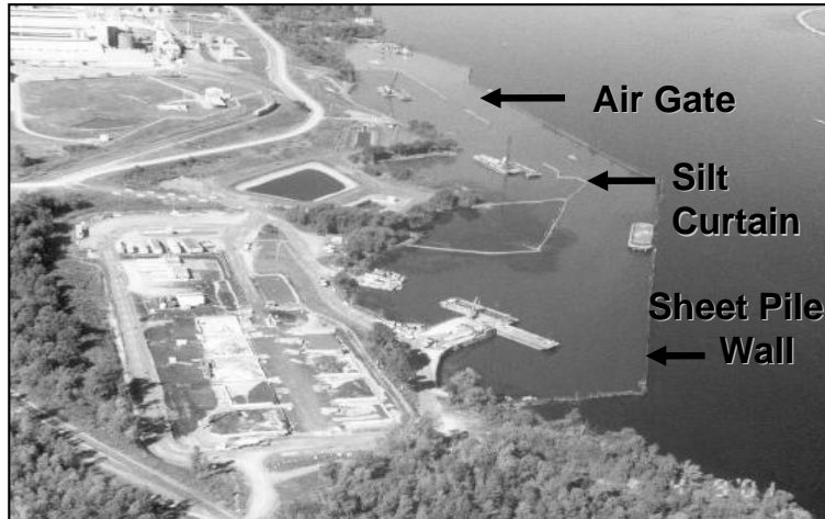
Environmental Dredging Control Measures and Management B-8
