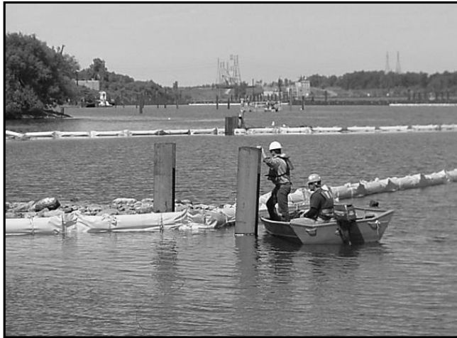
Environmental Dredging Control Measures and Management B-17
