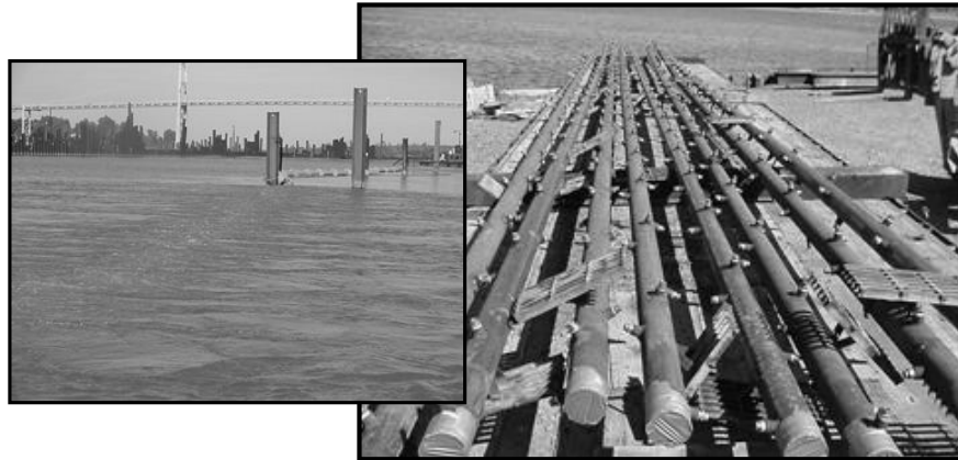
Environmental Dredging Control Measures and Management B-9
