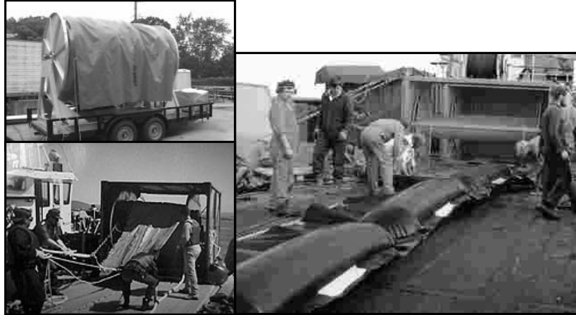
Environmental Dredging Control Measures and Management B-15
