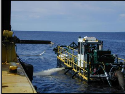
Manistique – outriggers used to control positioning of auger dredge
