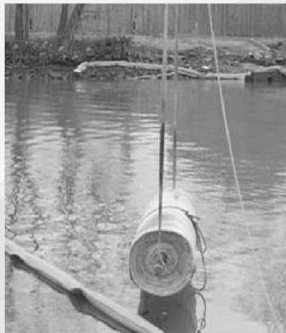
Placement on Subaqueous Sediment (courtesy of CETCO®)
