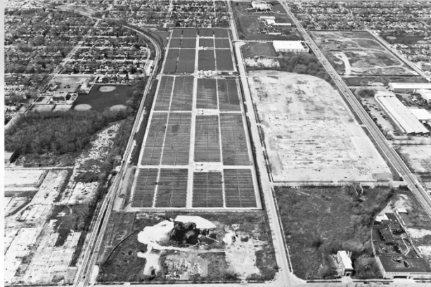
SunPower-Exelon City Solar , Chicago, Illinois Owner: Exelon Corporation Arch: SunPower Corporation General Contractor: SunPower Corporation Construction Manager: Turner / Riteway-Huggins Date: 04-10-10 View: W File# 19211-658 prt Photo By: McShane-Fleming Studios, Chicago
