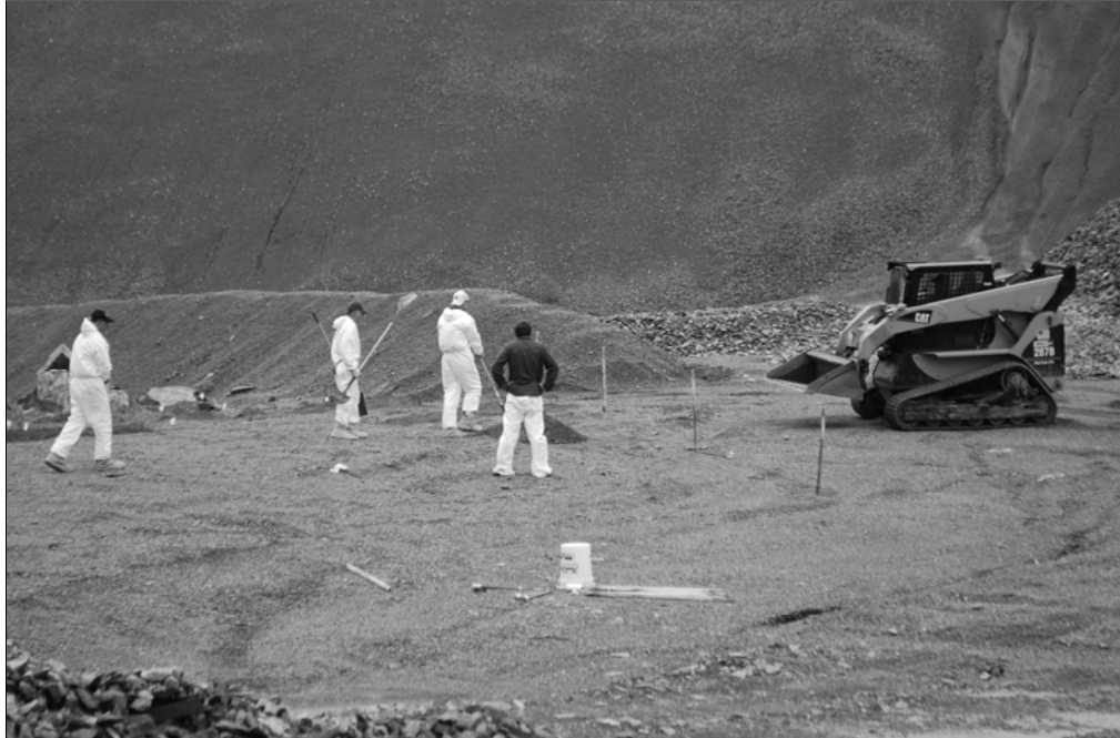
August 24, 2011: Applying the compost mixtures to test plots; compost was raked even, then seeded with crop mix. 97
