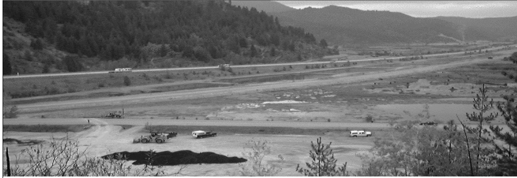
West Page Swamp prior to beginning treatment (10/7/98)
