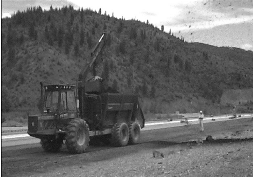
Aerospreader Applying Biosolids-Wood Ash Mixture at Bunker Hill 70
