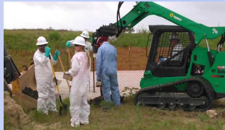
Pictured: TCT Construction (HDD and power pole installation)
