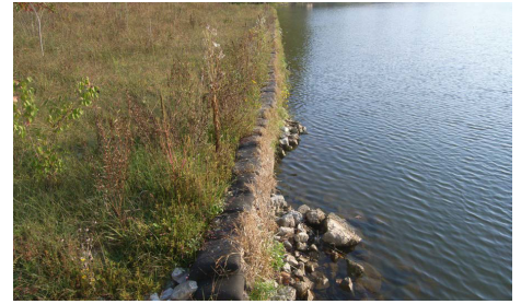
Revegetation of shoreline and wetland habitat used special native seed mixes, which corresponded to the topographic zones. Application of native seeds mixes took place at over 50 acres of the site. Several varieties of wetland shrubs were also planted.
