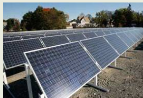
Fixed axis PV panels aligned to be south facing.
