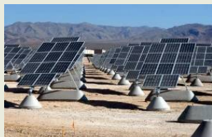
Tracking PV panels follow the sun to allow for increased solar capture.
