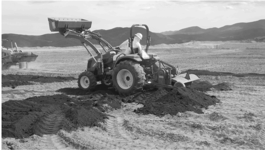
Mixing the compost into the tailings
