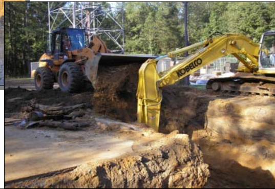
TCE Source Removal Adjacent to Radar Tower
