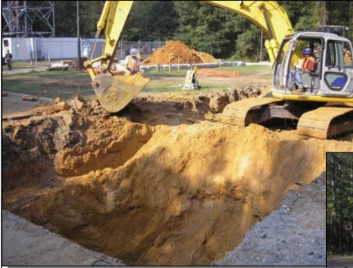
TCE Source Removal Adjacent to Radar Tower
