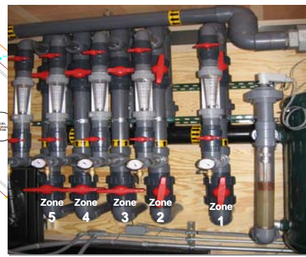
Trailer Manifold Piping
