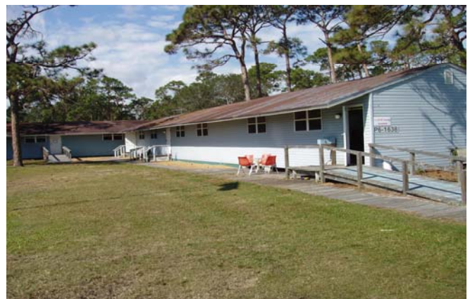
Figure 3-2. KARS Park recreation building.
