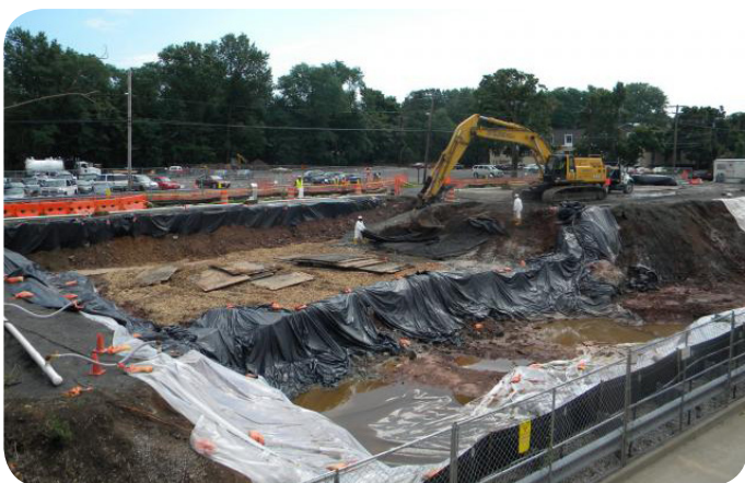
Soil piles are covered with plastic tarps during excavation.
