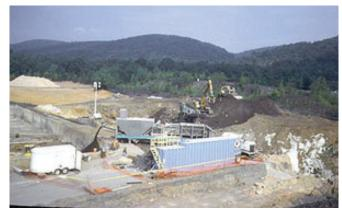
Contaminated soil mixed with cement in a pug mill is spread on the ground as pavement.
