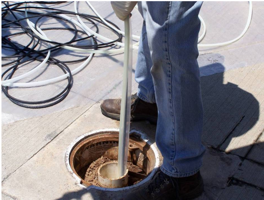
Figure 5-2. Polyethylene covering on electronic trigger line.
