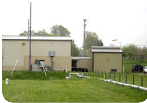
Groundwater Treatment Building
