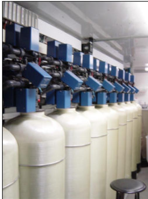
**Photograph 2: Interior of Basin Water high efficiency ion exchange system.**
