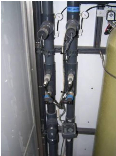
**Photograph 5: Inline pressure, flow, pH and conductivity meters.**
