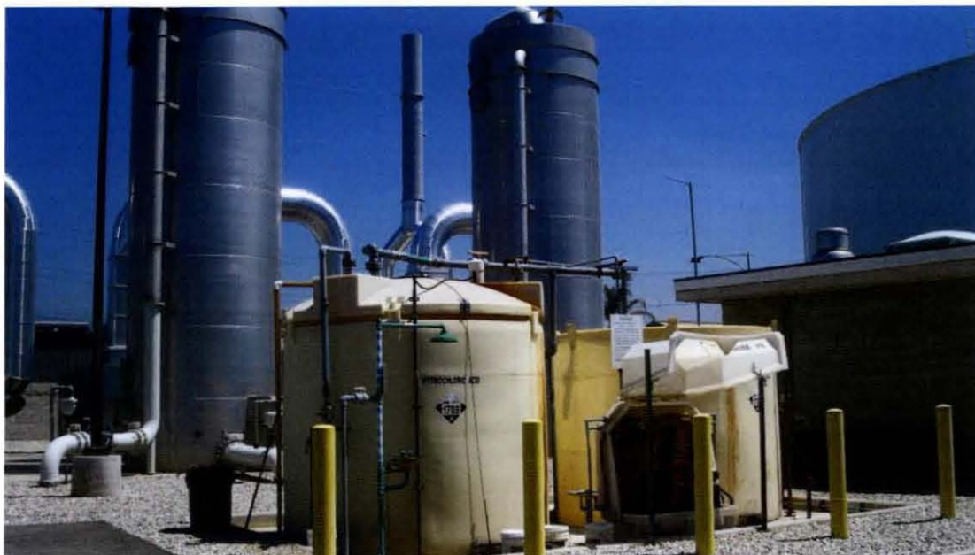
Figure 4. Tank Containing Food-Grade Hydrochloric Acid at the BPOU.
