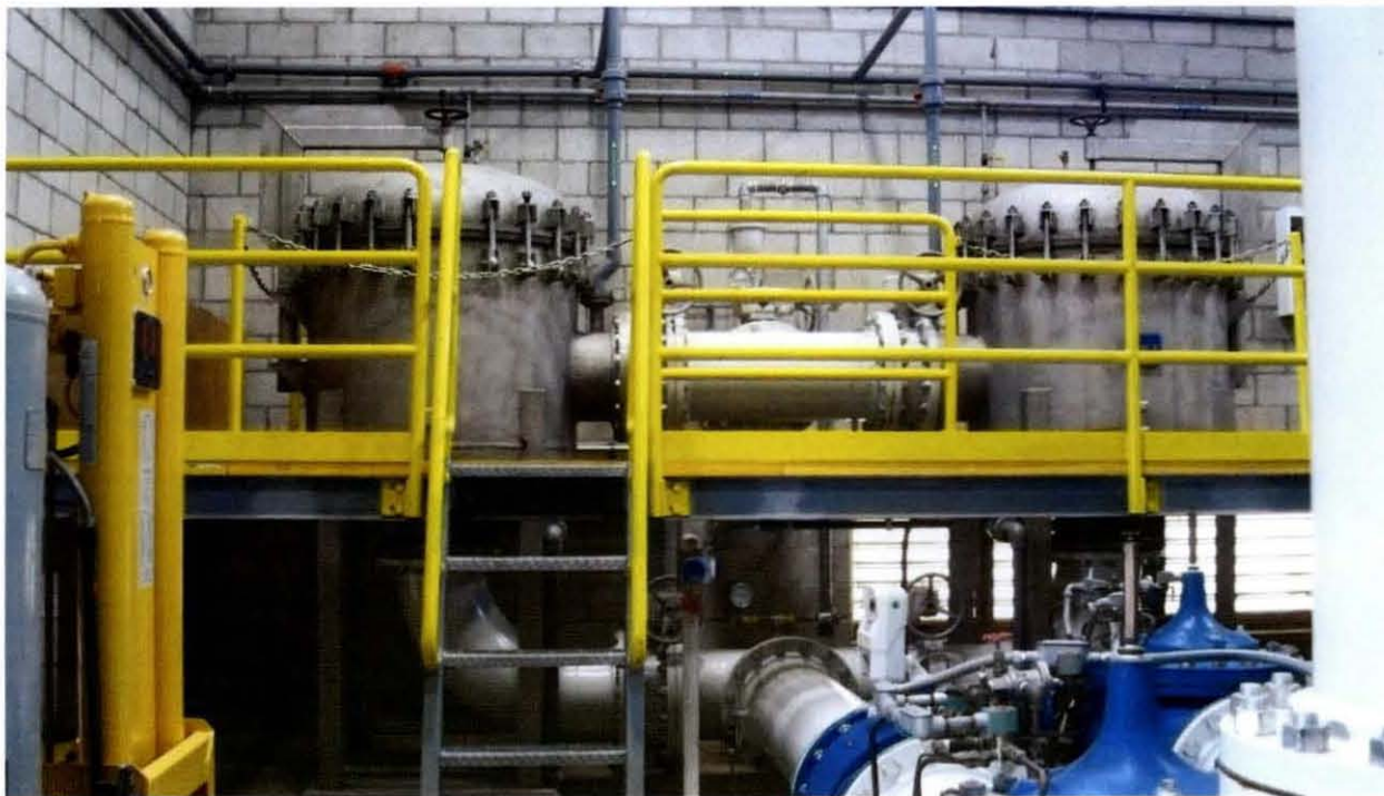
Figure 7. Particulate Filters for Pre-Treatment of Groundwater Prior to Entering Ion Exchange Resin Tanks at the BPOU.
