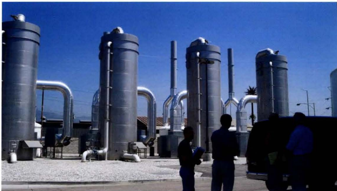
Figure 3. Baldwin Park Operable Unit Air Stripper/Vapor-Phase GAC Towers.
