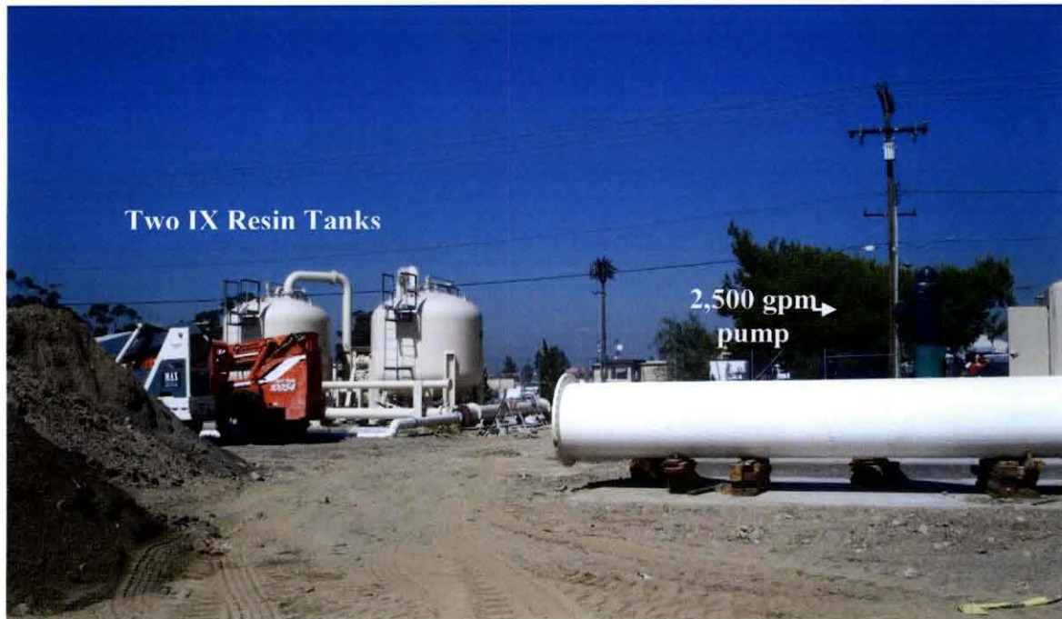
Figure 1. City of Rialto, CA Groundwater Treatment Demonstration System Integration Project under Construction.
