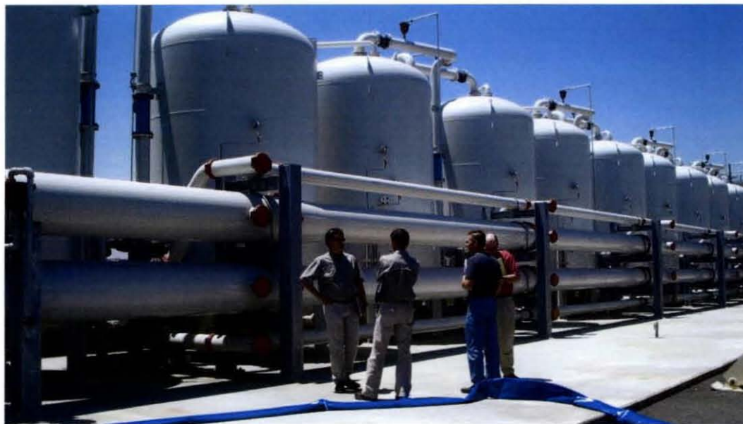
Figure 5. Liquid-Phase GAC Tanks for Removal of 1,2,3 Trichloropropane at the BPOU.
