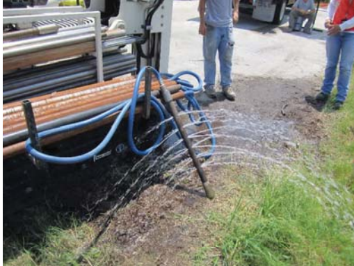
2 ft Injection tool during water test
