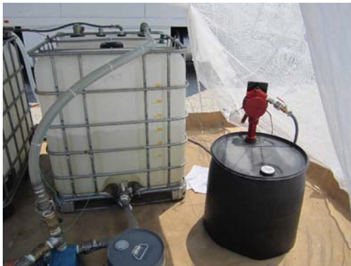
Bonding locations on drum pump and transfer pump
