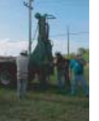
Figure 10: Injection tests with direct push rig
