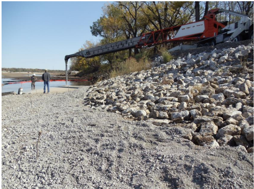
Below – View of Telebelt During Armor Stone Placement
