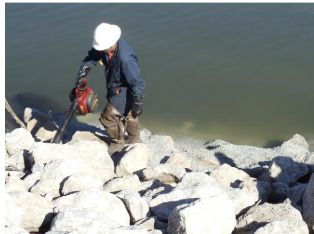
Left – Placement of AquaBlok Over Rip Rap Below - Using Blower to Distribute AquaBlok
