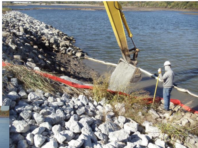
Left – Placement of AquaBlok Over Rip Rap Below - Using Blower to Distribute AquaBlok
