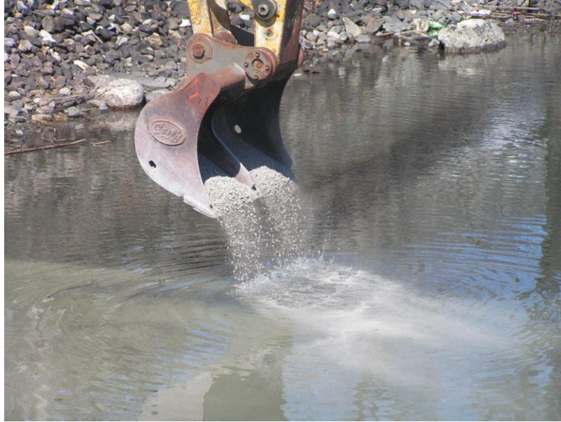
Placement of AquaBlok+ORGANOCLAY product through the water for treatment/adsorption of petroleum-based hydrocarbon contaminants
