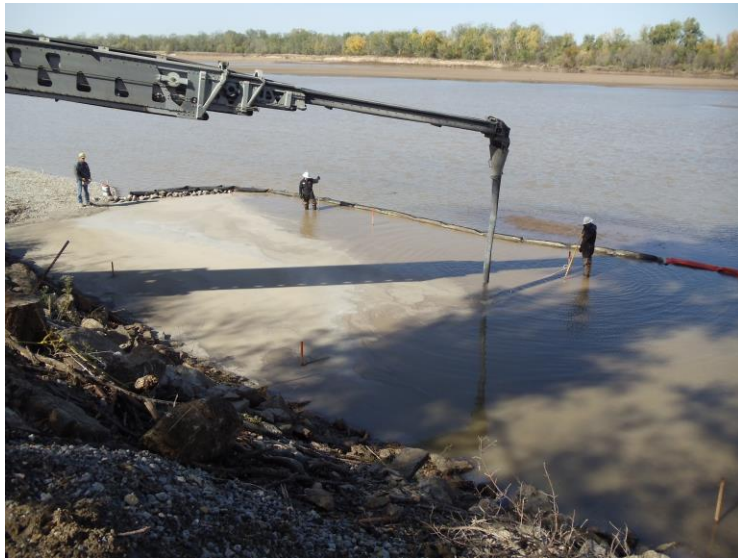
Above – Placement of AquaGate+Organoclay
