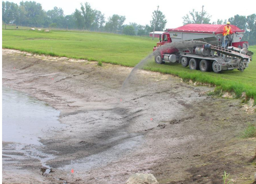
Overview of AquaGate+ORGANOCLAY being applied to pond basin
