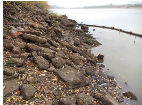
Above – Demo Debris Area - Before
