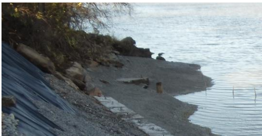
Above – Demo Debris Area - After
