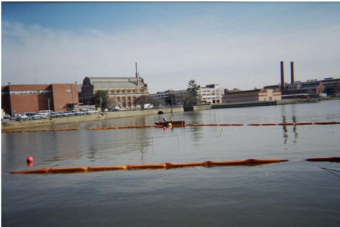
Figure 3-9. Silt Curtains Deployed Around Demonstration Area Capping Cells
