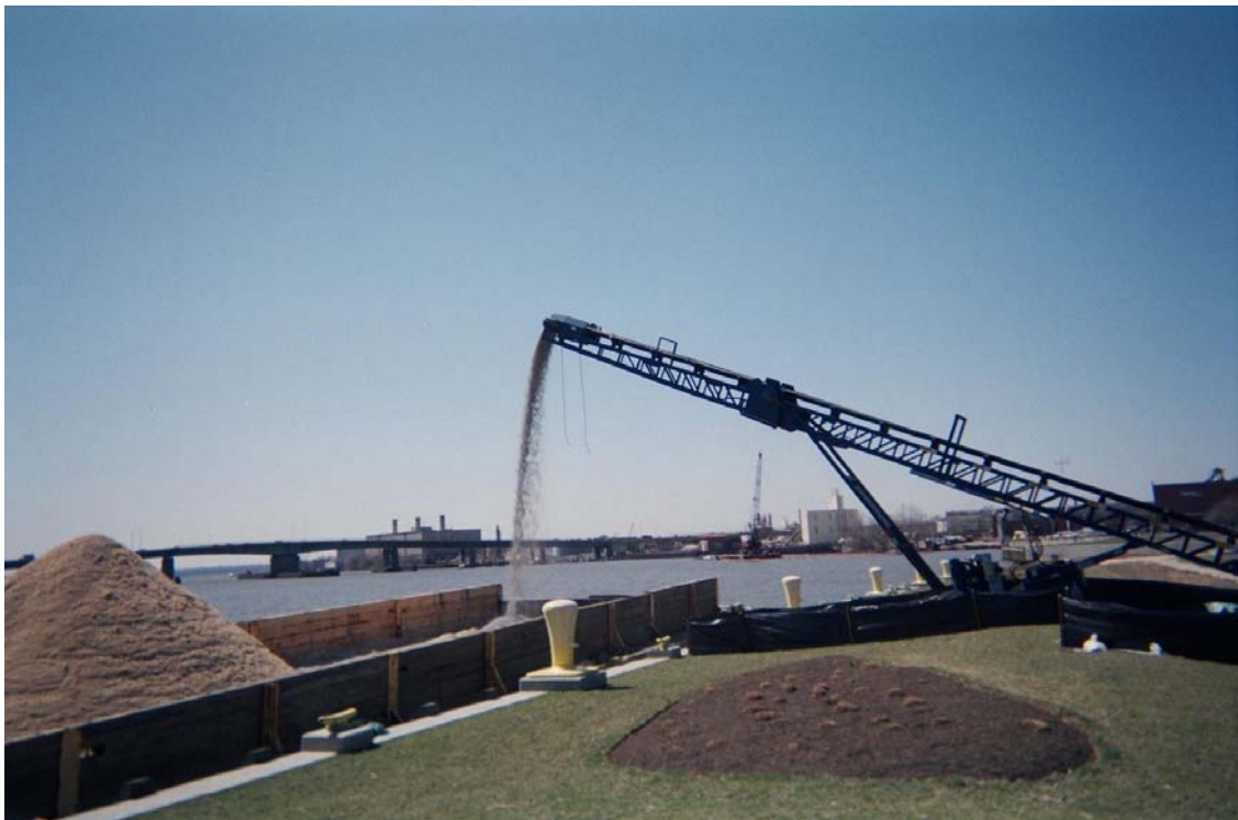
Figure 3-7. Transferring Cap Material to Barge Using Conveyor
