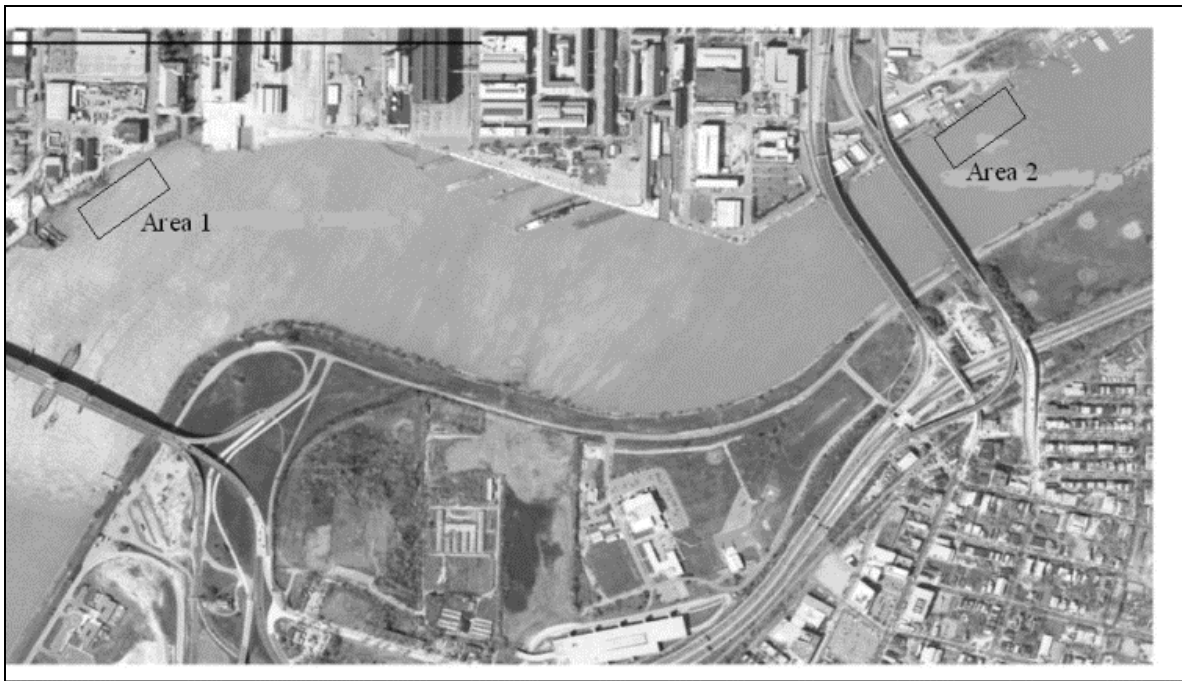
Figure 3-3. Aerial Image of Preliminary AquaBlok® SITE Demonstration Study Areas
