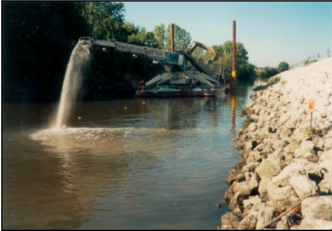
Figure 4-1. Typical Barge-Mounted Material Conveyor
