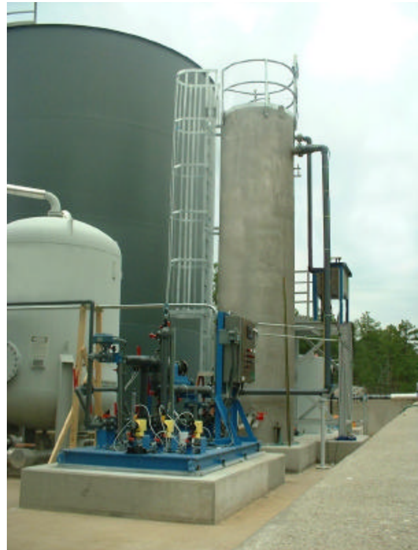
Figure 4. Full-scale FBR system at LHAAP during construction
