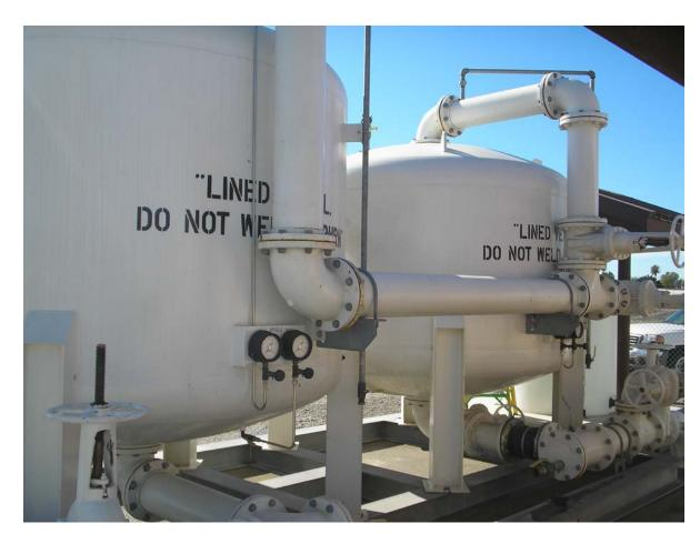
Figure 12. Face Piping and Well Connection – West Valley Water District
