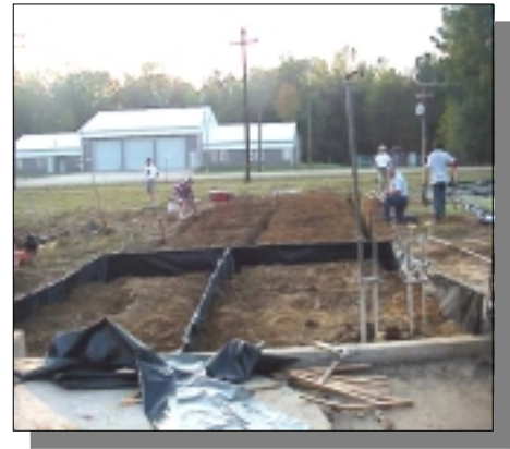
In situ bioremediation of perchlorate-contaminated soils at LHAAP
