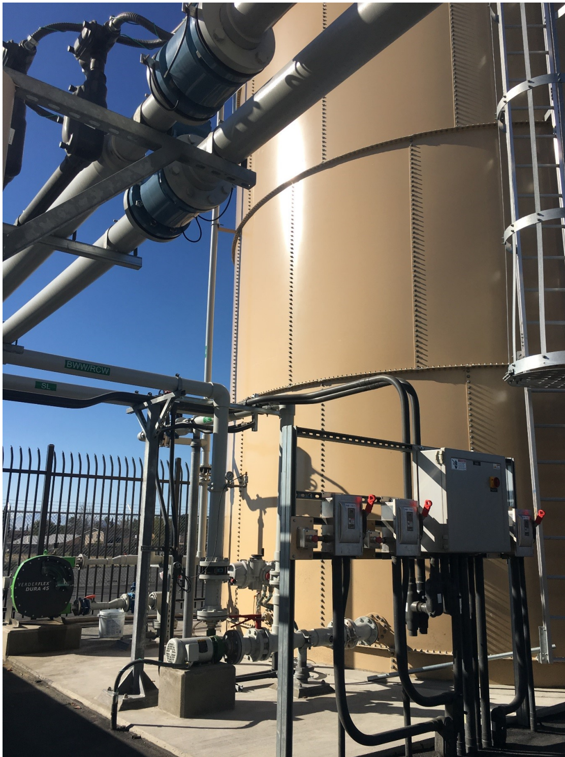
Figure 8 Completed Backwash Waste Tank
