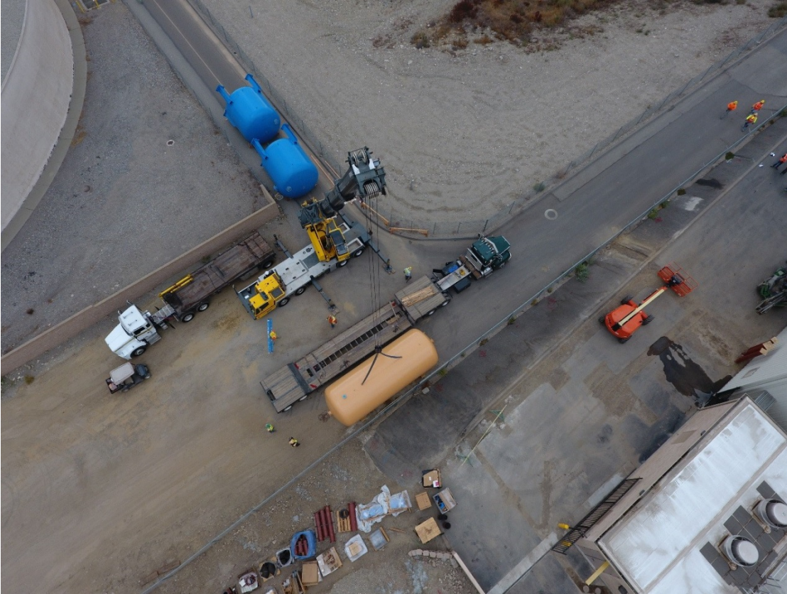
Figure 10 Delivery of the FXB Vessels and Treated Water Contact Tank
