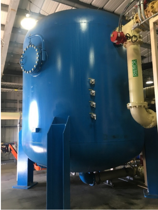
Figure 4 Completed Bioreactor
