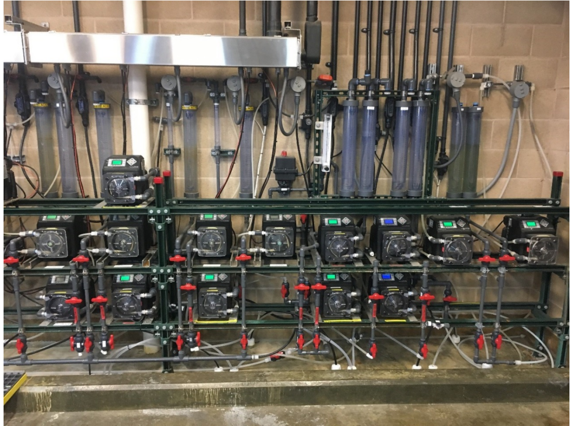
Figure 5 Chemical Feed Pumps
