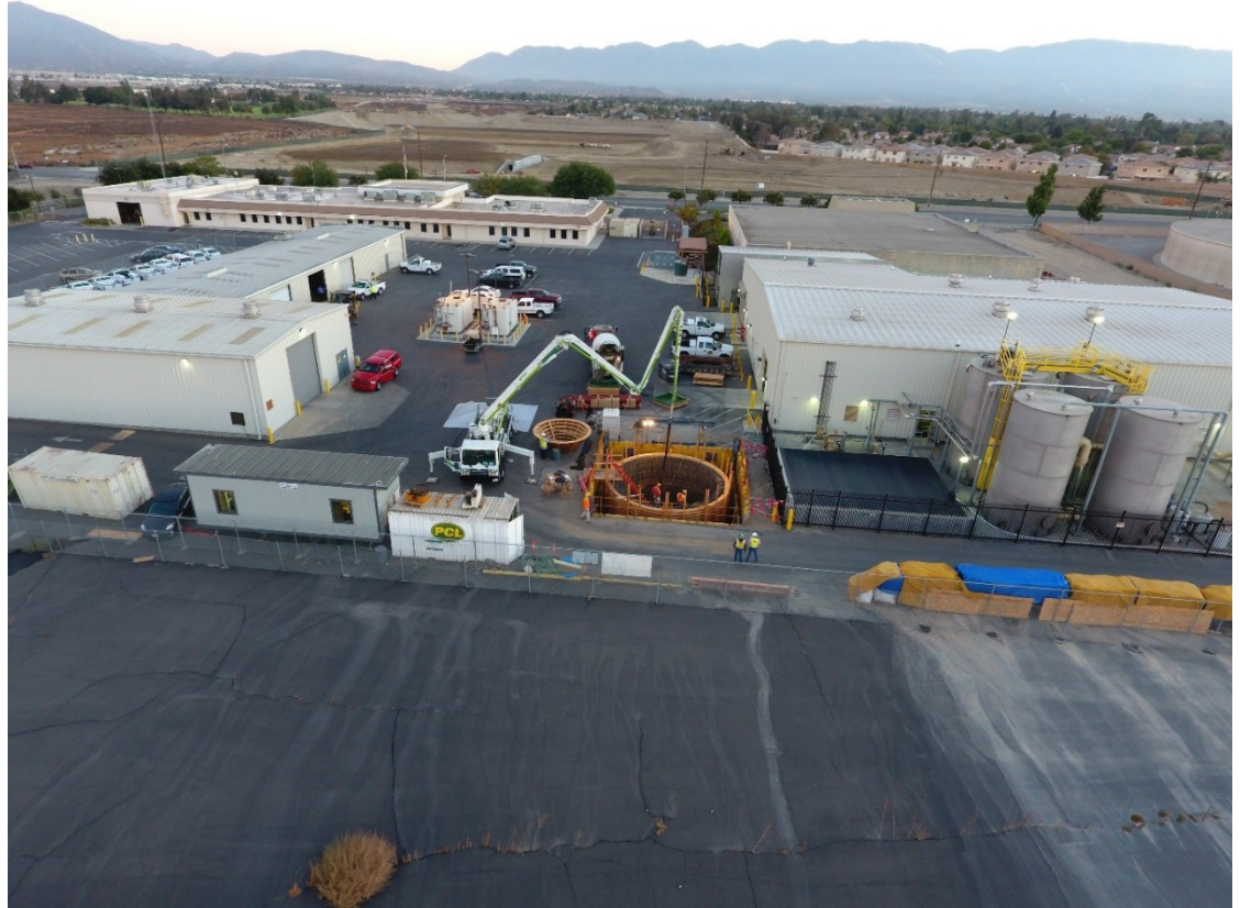
Figure 9 Construction of the Backwash Waste Tank
