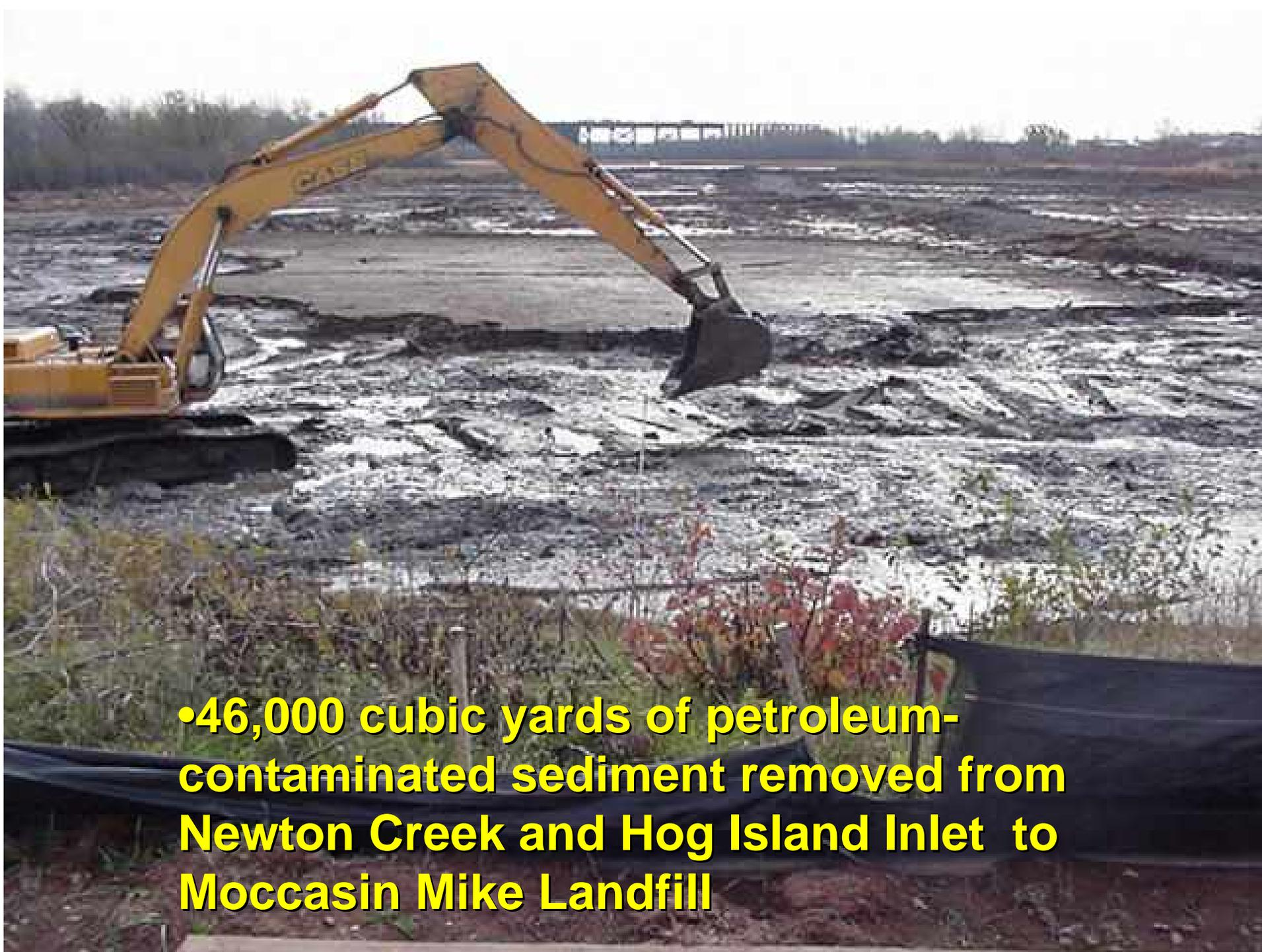
**•46,000 cubic yards of petroleum-contaminated sediment removed from Newton Creek and Hog Island Inlet to Moccasin Mike Landfill**
