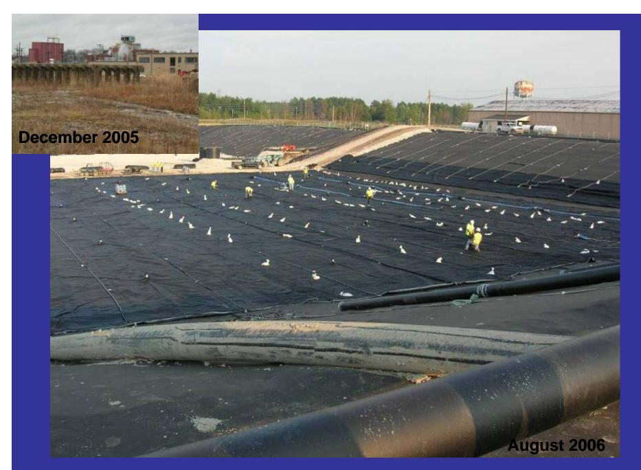
**CF** with geotube bags laid out in preparation for sediment dewatering
