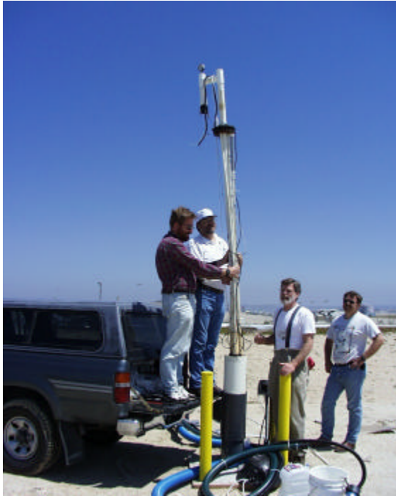
Photograph 19a: Well Air Unit
