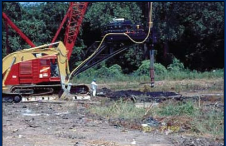
In-Situ Treatment of Sludge Pit Wastes at the South 8th Street Landfill Superfund Site in West Memphis, Arkansas
