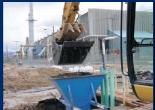
Backfilling of Trench with Granular Iron
