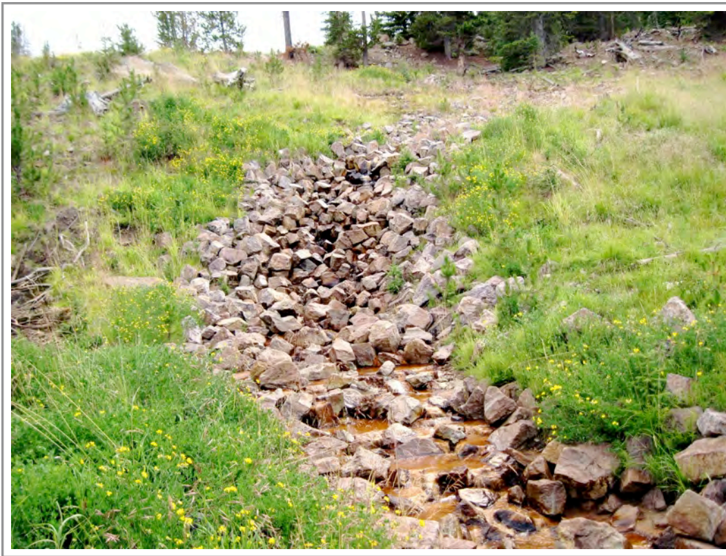
Photo 12. Constructed channel containing the acid mine drainage from the adit just above the confluence with Jill Creek. Notice the color of the water
