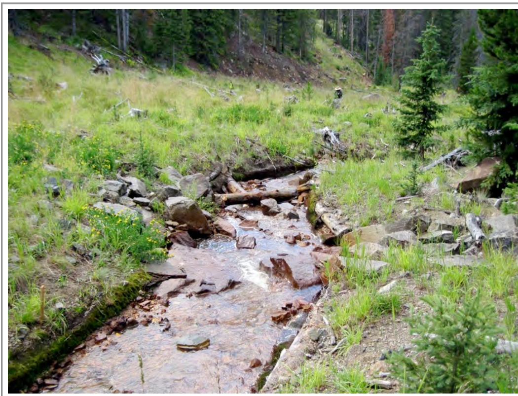
Photo 30. Looking downstream on Lower Jill Creek showing engineered streambanks, drop structures, and stained streambed
