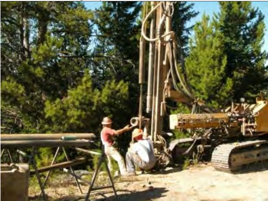
Drill rig set up and well installation at BM-MW-3
