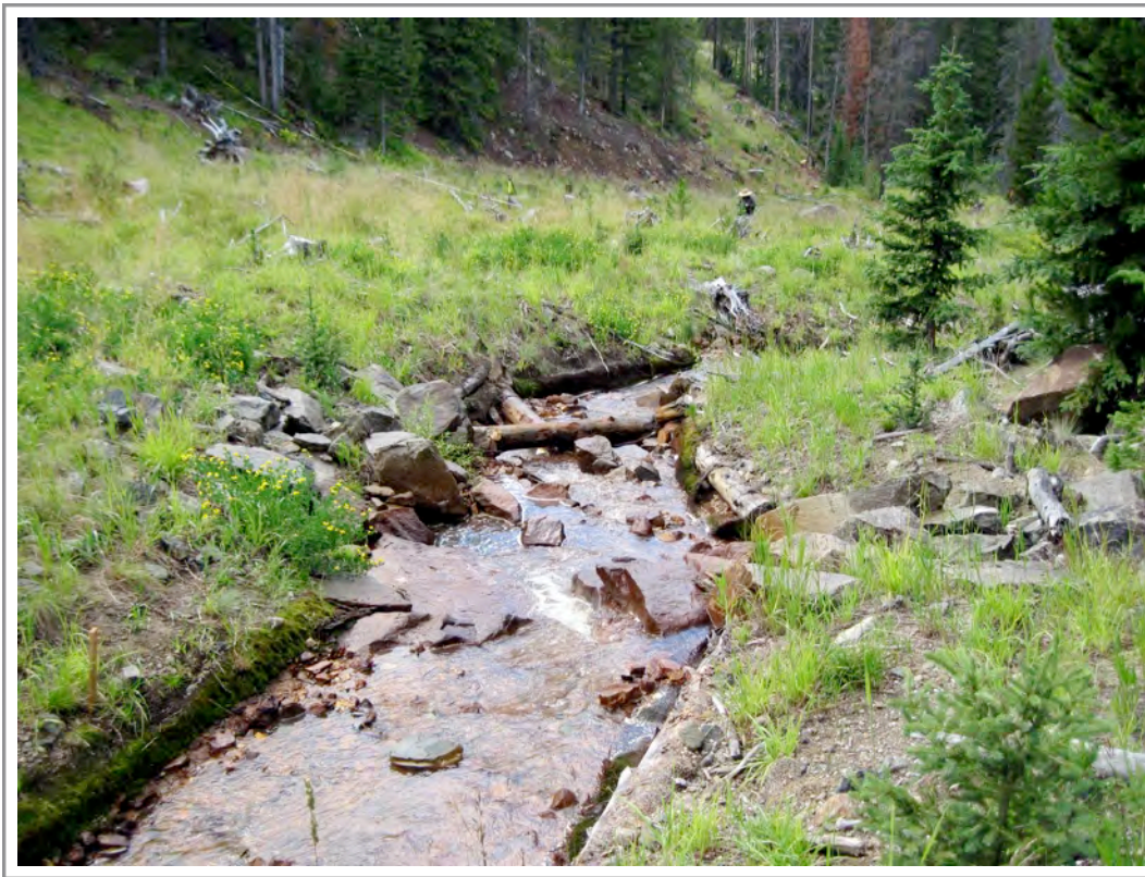
Photo 16. Downstream of confluence showing engineered streambanks, drop structures, and stained streambed
