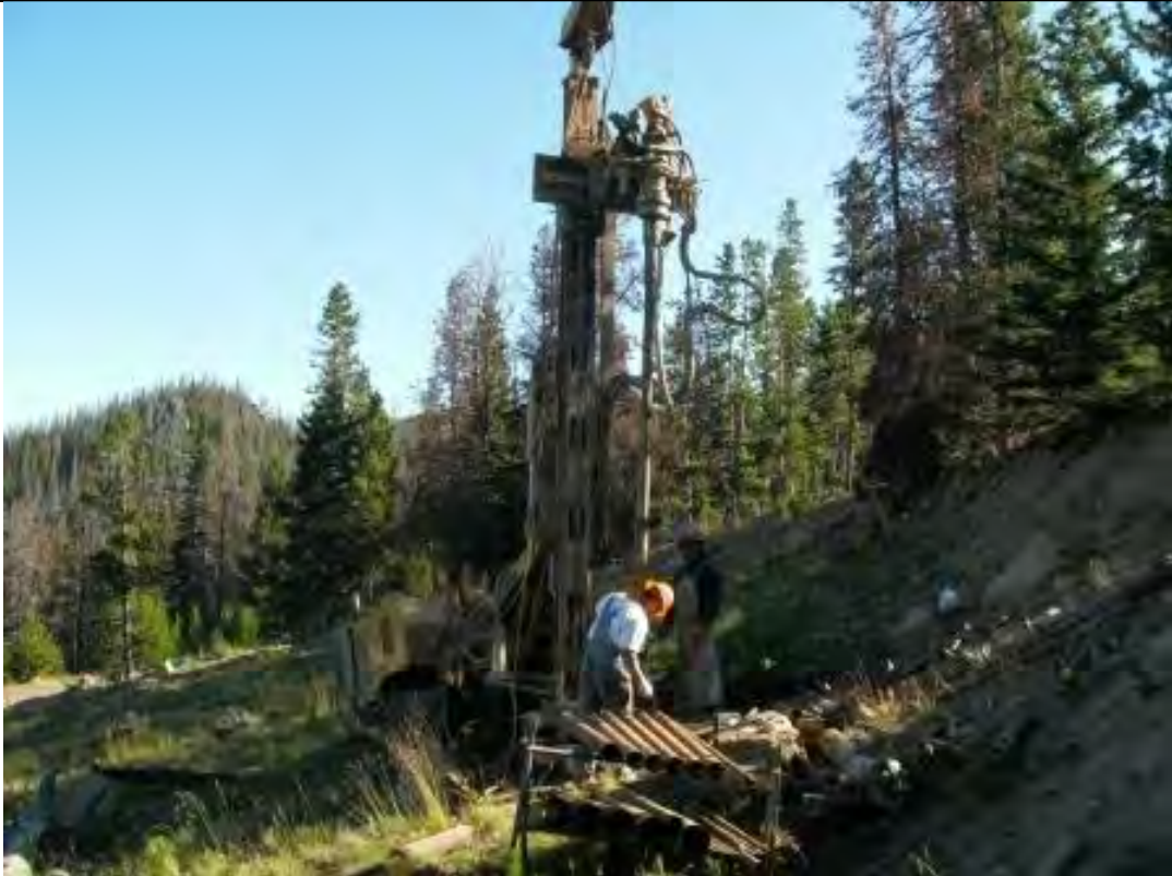
Drill rig set up and well installation at BM-MW-4
