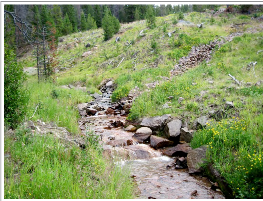
Photo 15. Looking upstream of Jill Creek showing the confluence with the adit. The streambanks are engineered with rock, logs, and coir fabric
