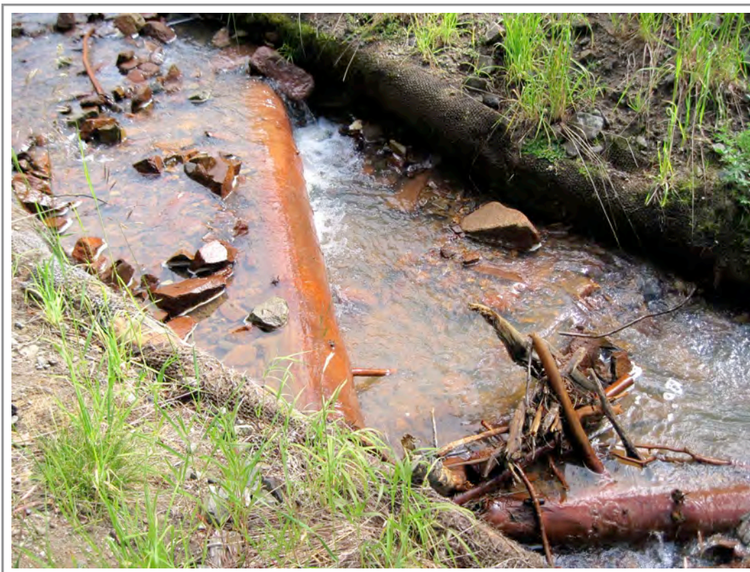
Photo 19. Notice the reconstructed streambanks and stream channel with energy-dissipating log drop structures. Notice the cloudy water and stained streambed and log structures
