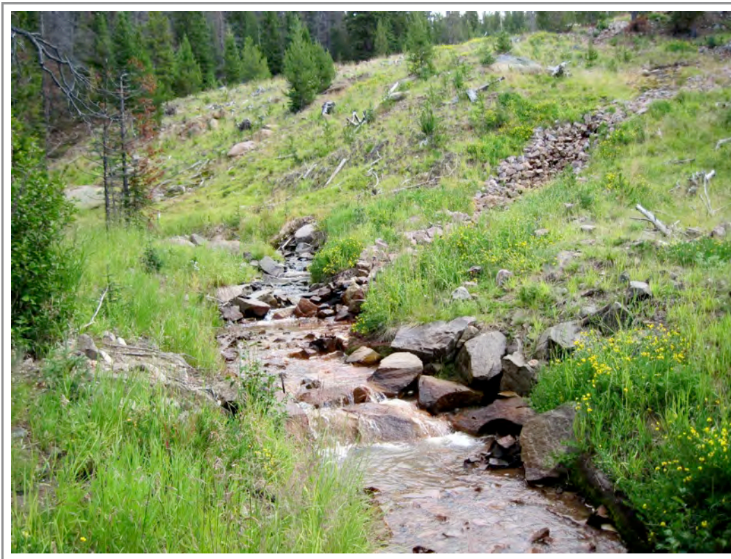
Photo 29. Looking upstream on Lower Jill Creek showing the confluence with the adit. The streambanks are engineered with rock, logs, and coir fabric
