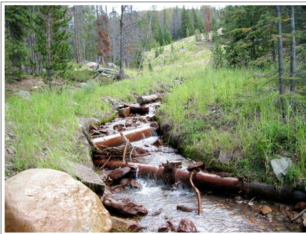
Photo 23. Lower end of the study area showing the energy dissipating drop structures placed throughout the stream channel
