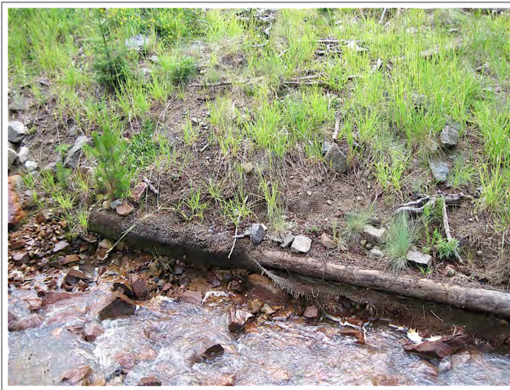
Photo 18. Reconstructed streambank (2001-2002) with logs and coir fabric
