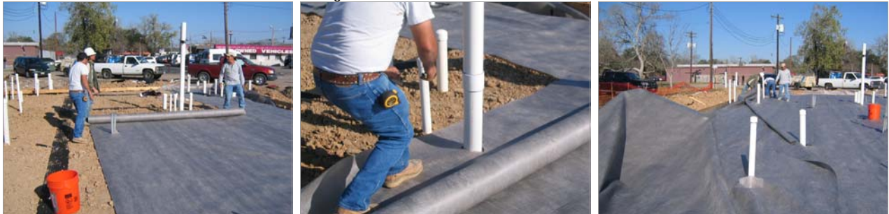
STEP 2: LIQUID BOOT® Base Fabric T-60 being laid out.
