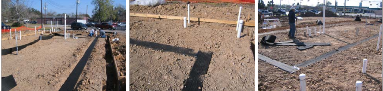
STEP 1: LIQUID BOOT® GeoVent being installed for the passive venting layer
