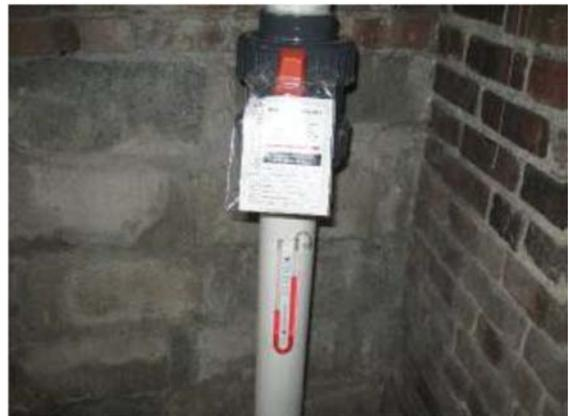
**Figure 3-12. Photos of mitigation system: (left) SSD blower and stack on northeast corner of duplex; (right) SSD extraction point showing valve and U-tube manometer.**
