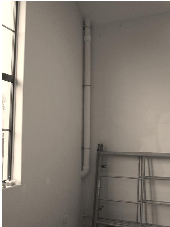
Figure 16: System Nine pipe routed through interior to roof
