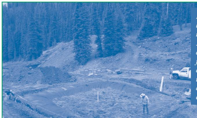
**Figure 2.** The biochemical reactor occupies a 35- by 35-foot area approximately 200 feet from the mine adit and 25 feet upgradient of the aerobic polishing cell.
