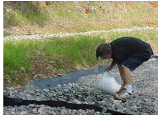
Figure 3. Inoculation of bacteria solution into a port extending into limestone emplaced at the Kimble Creek site
