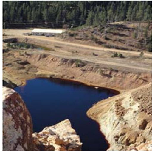
Figure 5. One of two onsite pits holding high-sulfate water at the Gilt Edge Mine site
