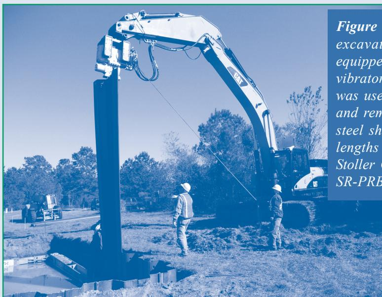
*Figure 2. An excavator equipped with a vibrator hammer was used to install and remove the steel sheets along lengths of the Stoller Chemical SR-PRB.*
